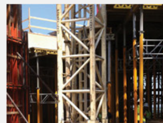
C&C enlisted one MX 34/38Z placing boom with lattice tower for the project.
