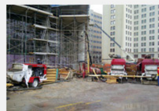
C&C Concrete Pumping, Inc. enlisted two of their BSA 14000 HP-D 8
