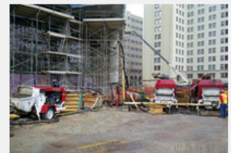
C&C Concrete Pumping, Inc. enlisted two of their BSA 14000 HP-D 8
