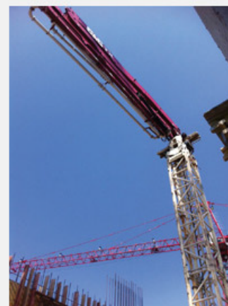
C&C enlisted one MX 34/38Z placing boom with lattice tower for the project.
