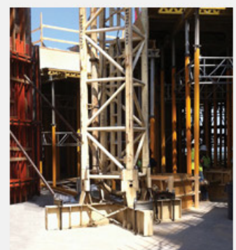
On the roof of the building, C&C installed a
